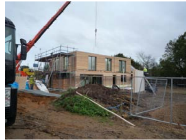
Construction under way
