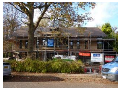
Day 5 of construction – finished!
