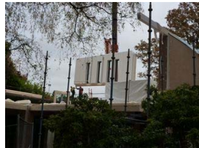
A first floor wall being placed
