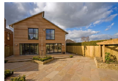
View of Rear
